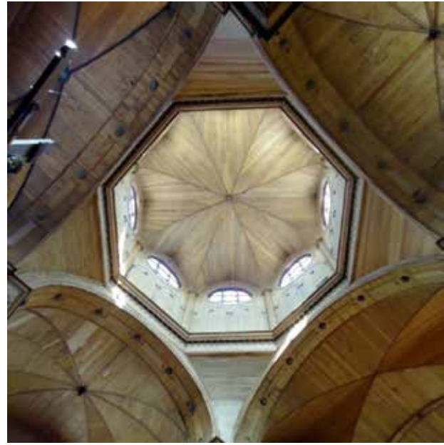
Figure 3. Octagonal dome of the Church of San Francisco de Castro in Chiloé, Chile Source: photograph by authors.
